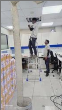
industrial air conditioning maintenance service and repair
