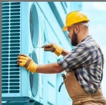
Split AC Repair
