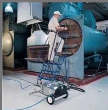
Condenser Cleaning Service
