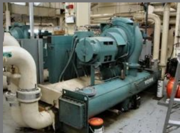
Water Chilling Plant Repairing Services
