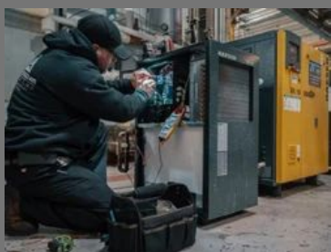
Screw Air Compressor Repairing Service
