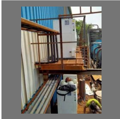
Ductable Ac Unit Installation
