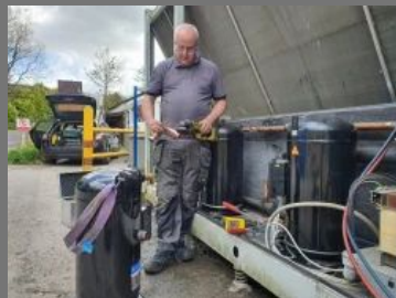
Water Chilling Plant Repair And Services
